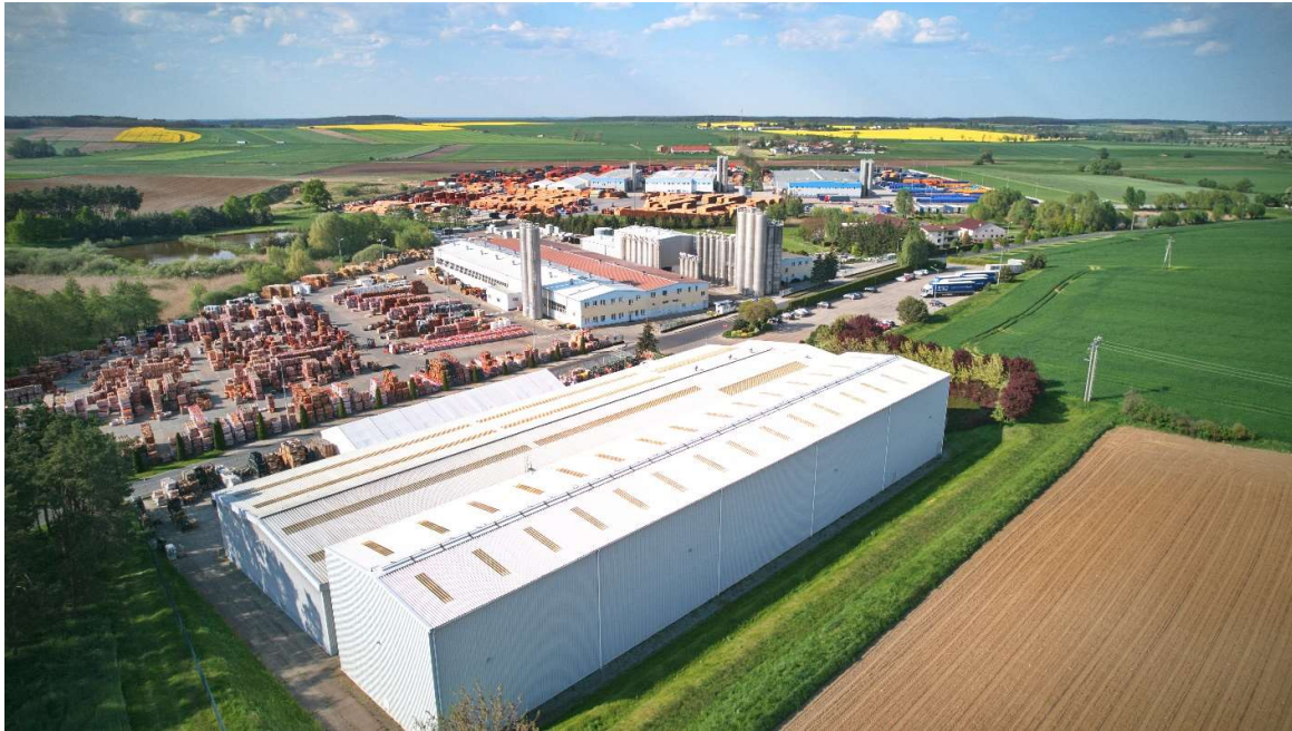
Figure 1. Production plant in Malewo.
