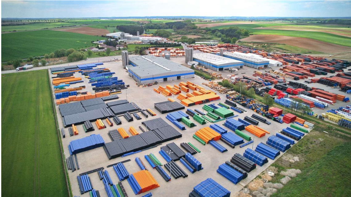
Figure 1. Production plant in Malewo.
