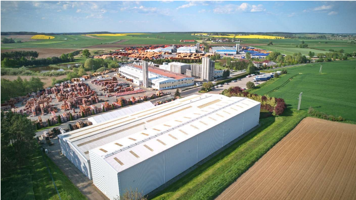
Figure 1. Production plant in Malewo.
