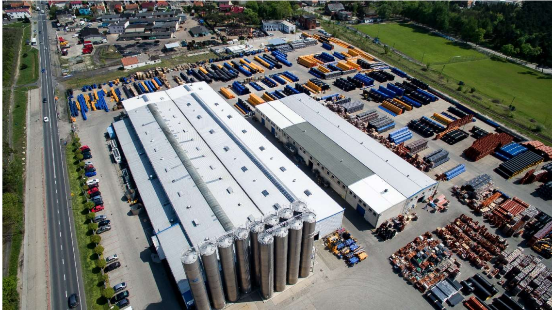
Figure 1. Production plant in Piaski.
