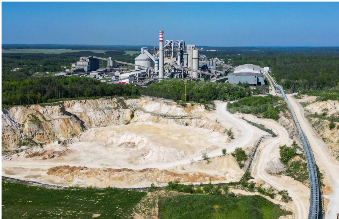
Figure 1. View on Cementownia Warta S.A. and Mining Plant „Działoszyn”, A lump in the excavation of the deposit „Niwiska Górne – Grądy.
