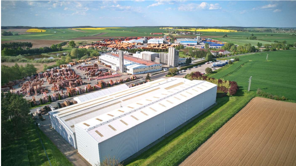
Figure 1. Production plant in Malewo.
